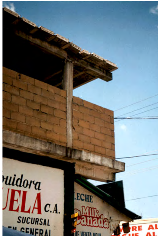
image 3: concrete frame construction
