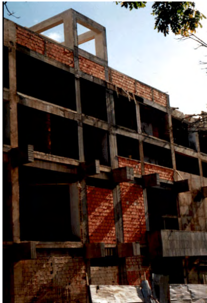
image 7: concrete frame construction
